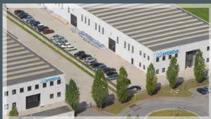
Sferova Headquarters and main production plant is located approx. 30 km North-East of Milan and covers a total area of 22.000 square meters.
