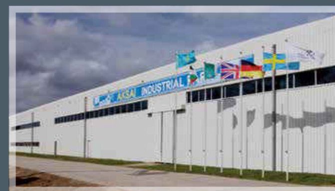
Sferova was selected to take part in the Aksai Industrial Park (AIP) Sferova Kazakhstan can manage assembling, testing, painting and after sales activities.
